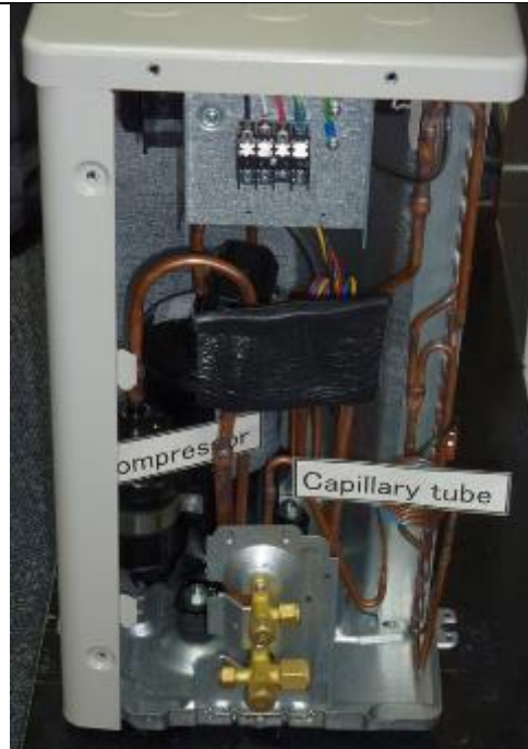
Figure 25: Example of outdoor unit showing service valves and interior components (Source: HEAT GmbH)
