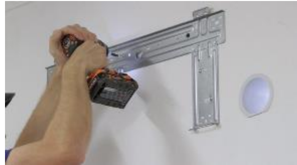
Figure 15: Mounting the installation bracket (Source: http://aroundhomediy.com )
