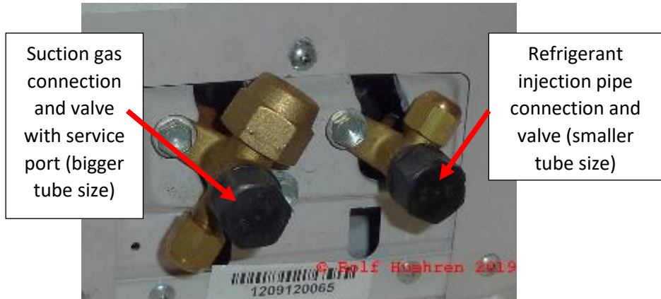
Figure 22: Example of outdoor unit showing typical refrigerant pipe connections (Source: HEAT GmbH)
