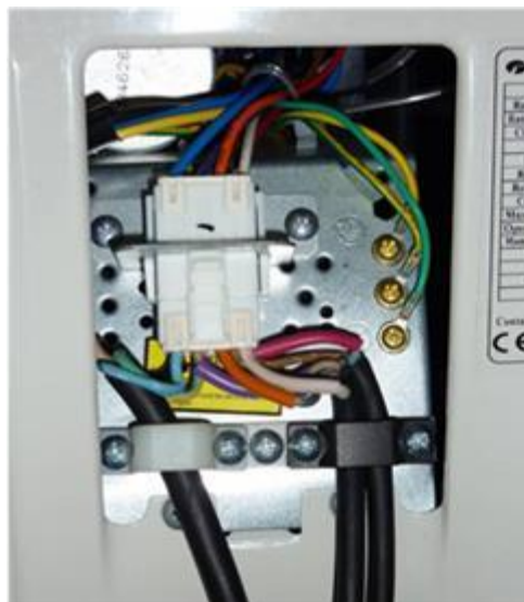
Figure 26: Examples of adequate electrical connections in outdoor unit (left) and indoor unit (right) (Source: HEAT GmbH)
