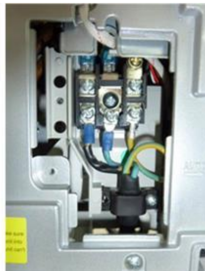
Figure 26: Examples of adequate electrical connections in outdoor unit (left) and indoor unit (right) (Source: HEAT GmbH)
