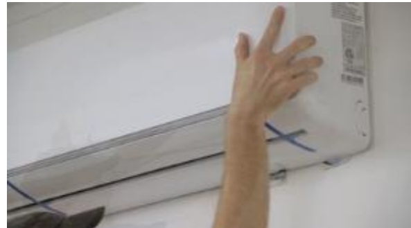
Figure 18: Indoor unit goes towards bracket, covering the hole through the wall (Source: http://aroundhomediy.com )
