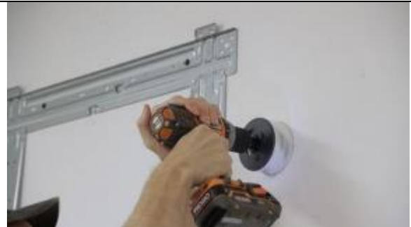
Figure 17: Drilling the tubing hole through the wall (Source: http://aroundhomediy.com )
