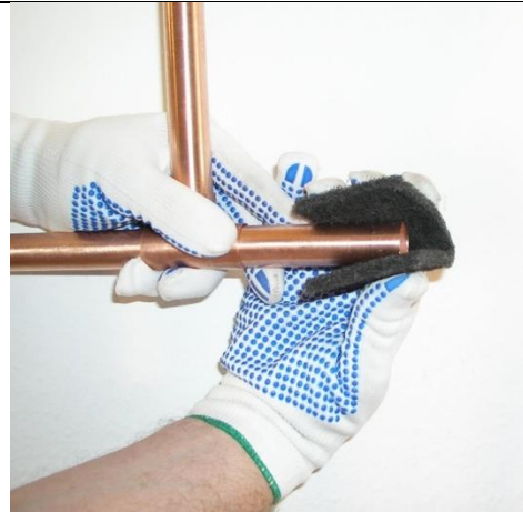
Figure 4-9: Assembly cleaning before brazing (Source: HEAT GmbH)
