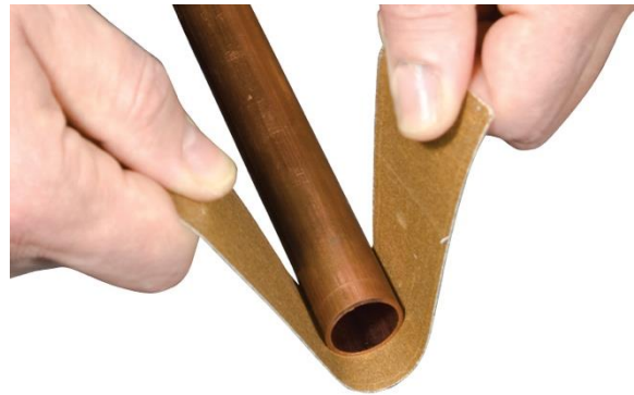
Figure 2-11: Use of sand paper at copper pipes (Source: HEAT GmbH)
