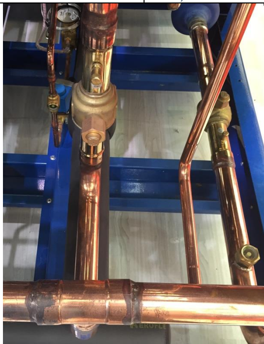
Figure 4-20: Example of bad brazing joint (Source: HEAT GmbH)
