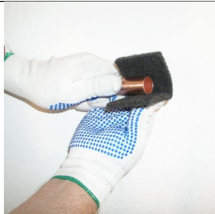
Figure 4-6: Outer area cleaning with cleaning pad or wire brush (Source: HEAT GmbH)
