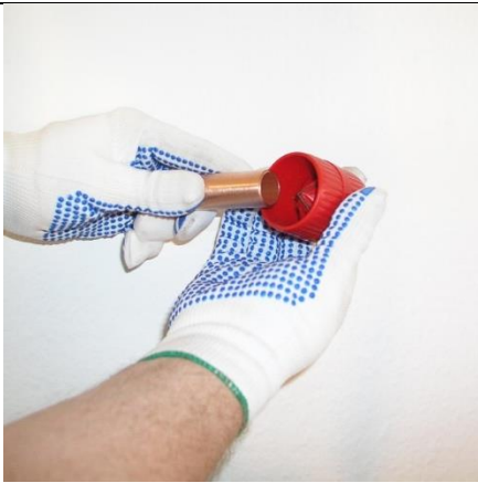
Figure 4-5: Deburring with “inner and outer deburrer” (Source: HEAT GmbH)
