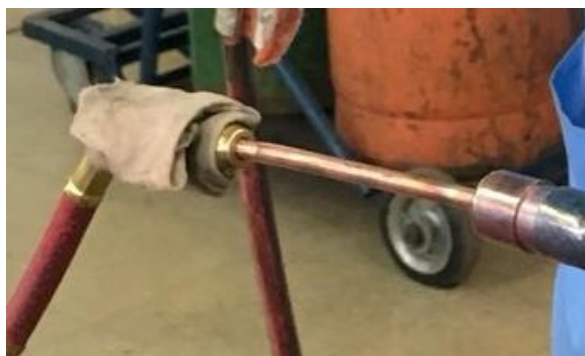
Figure 4-2: Schrader valve at a prepared copper cap for tubing connection (OFDN) (Source: HEAT GmbH)
