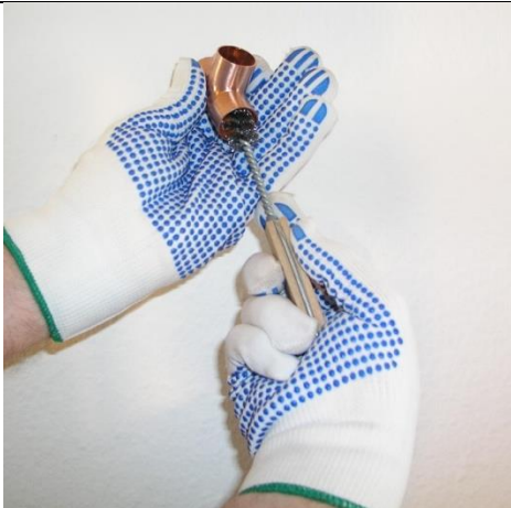
Figure 4-8: Inner cleaning with wire brush (Source: HEAT GmbH)
