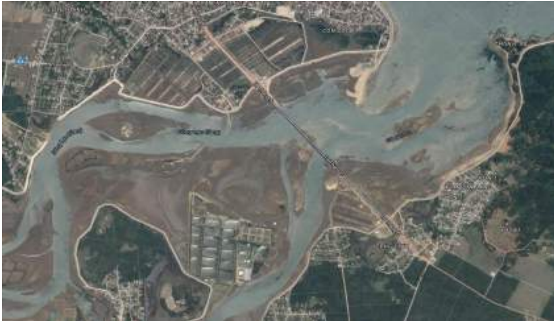
Photo 0.8: Cua Nhuong Bridge - 1,390 m long, built 2010-2015, second longest bridge in Central Vietnam. Google Earth, Aug 2014
